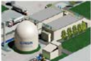
Anaerobic Digestion Facility
