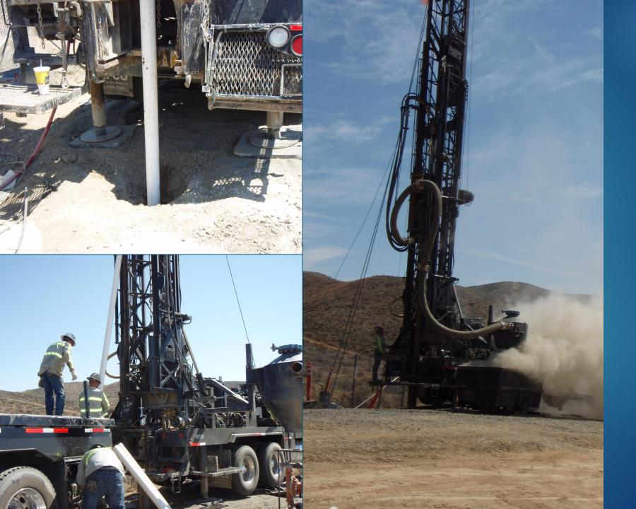
Groundwater Monitoring Well Construction
