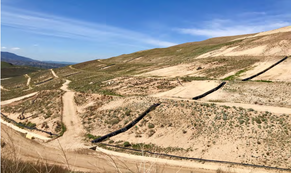
Photograph 2. Proposed irrigation areas on the right and densely vegetated areas on the left of the landfill slope.
