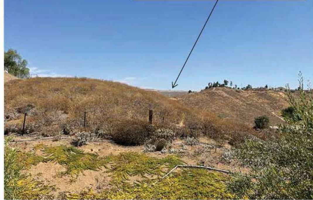
View of the Landfill from the Terramor Community
