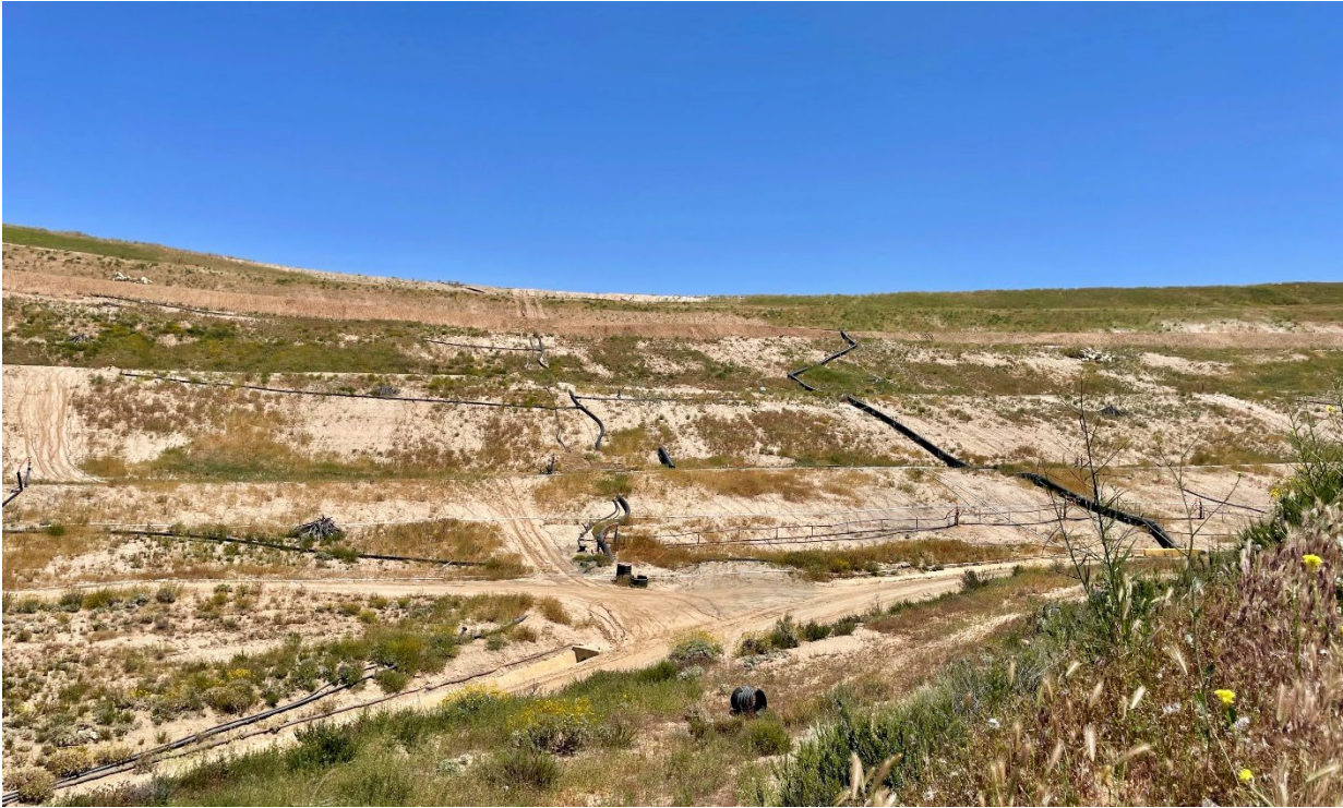
Photograph 10. The Phase C1 repair area shows plant growth, April 2023.
