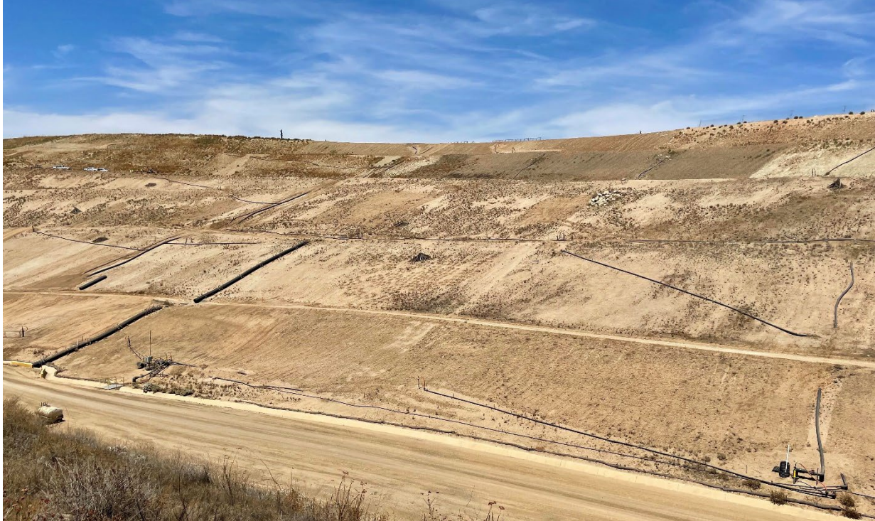
Photograph 11. Three slopes of Phase C1, July 2022.
