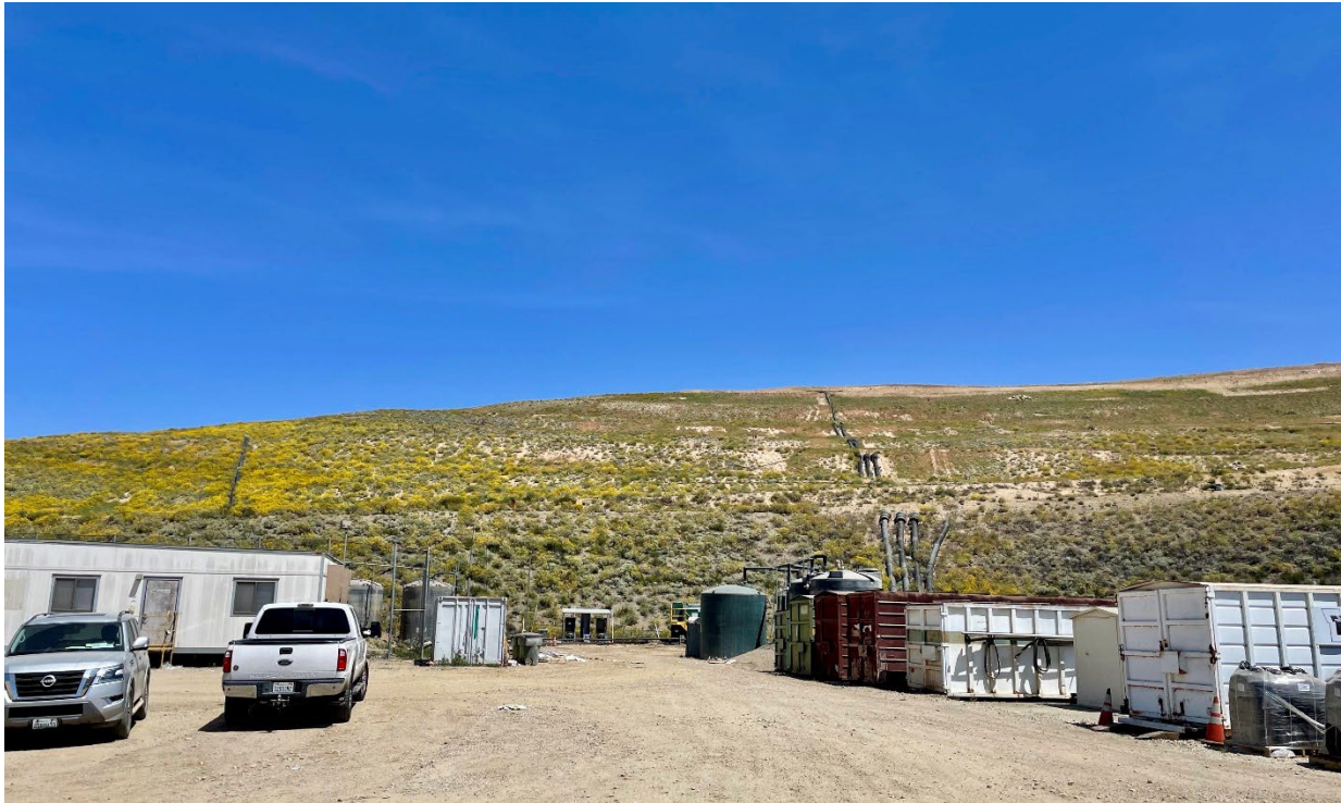
Photograph 6. The same pipes as Photograph 5 at the west end of the landfill, April 27, 2023.
